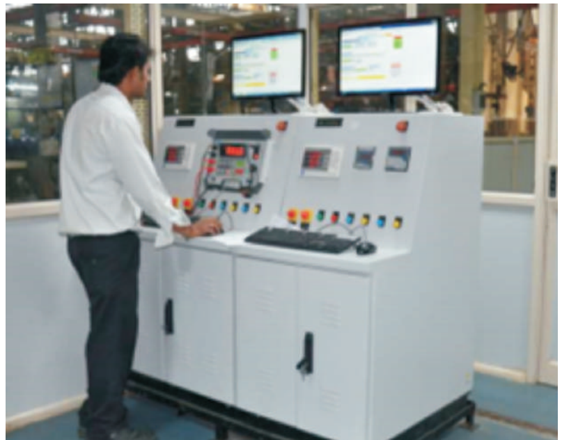
SCADA Test Facility
