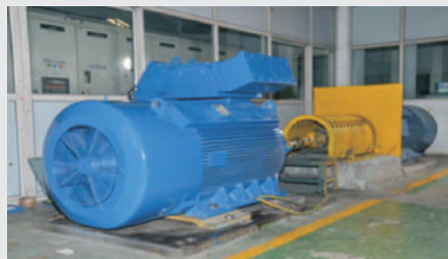
Large Motor Test Facility
